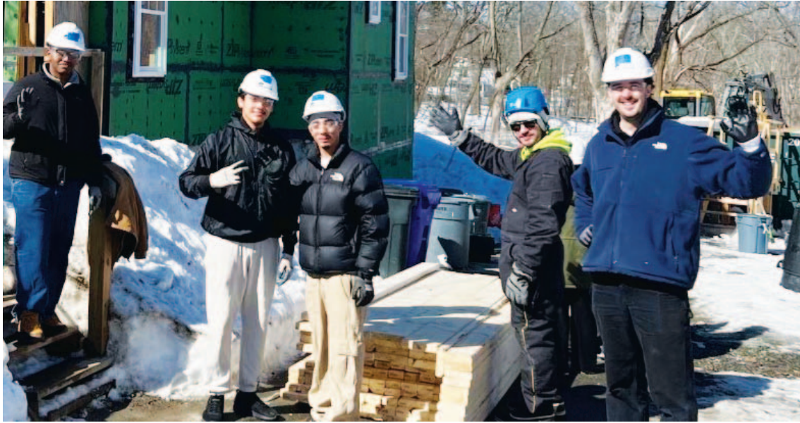
LANA members are gearing up to help build the four new affordable condo units at 104-108 Walter St.
