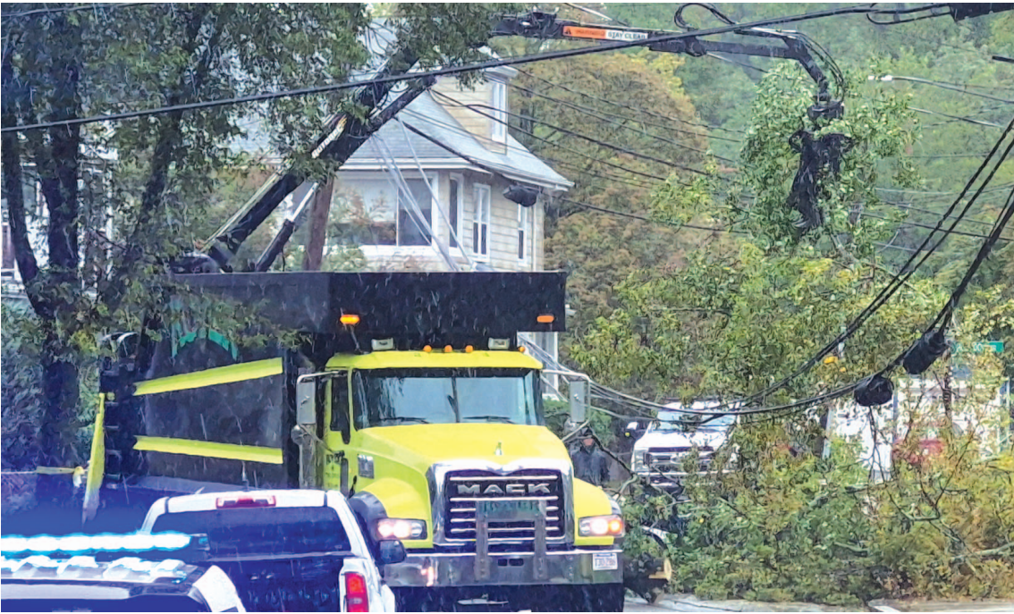
Trees caused damage all over the city, but crews were quick to pick them up, like here on Midvale Road off Corey Street.
